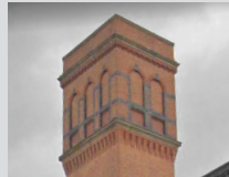
Water Tank Tower
