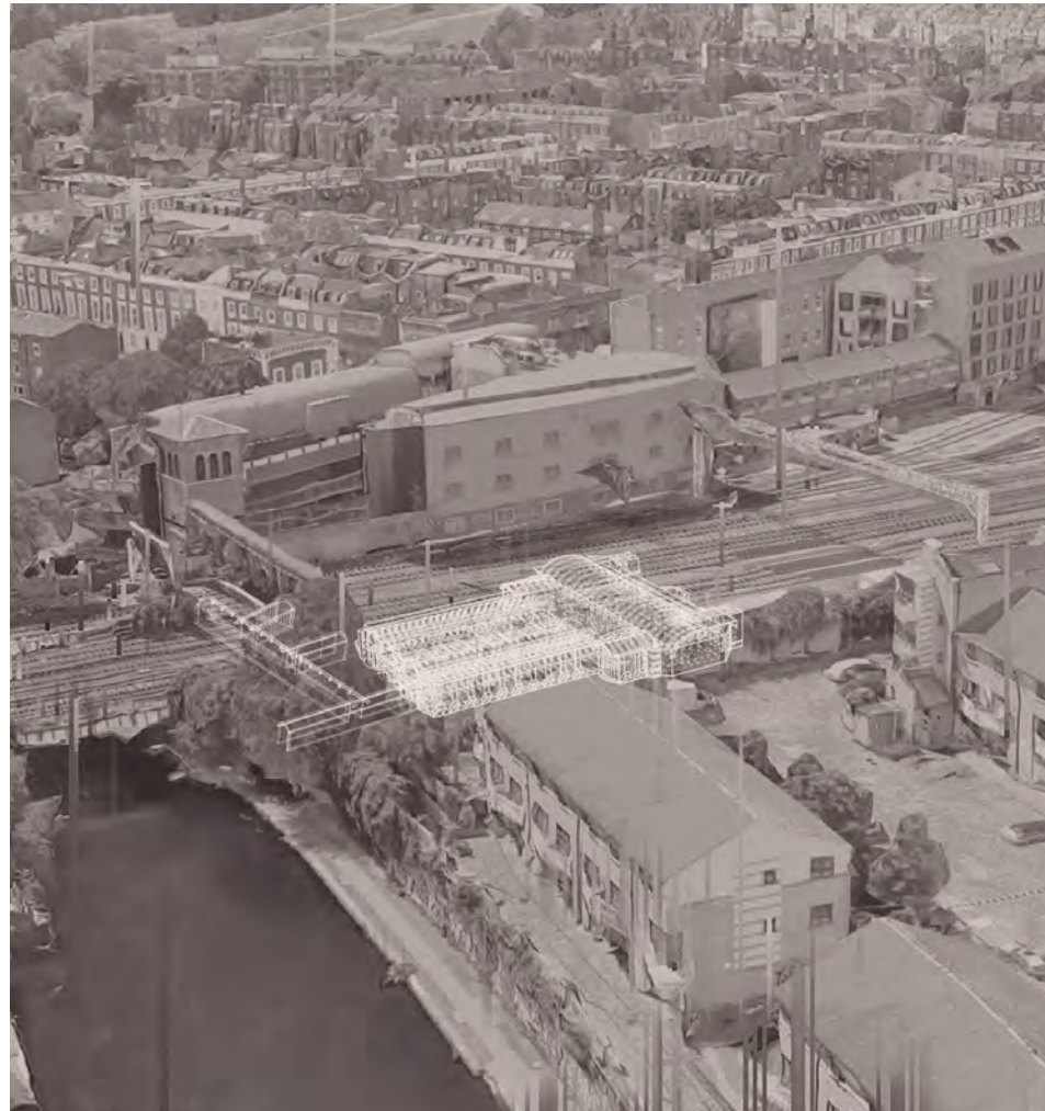
It located under the main line north of Fitzroy Bridge.
