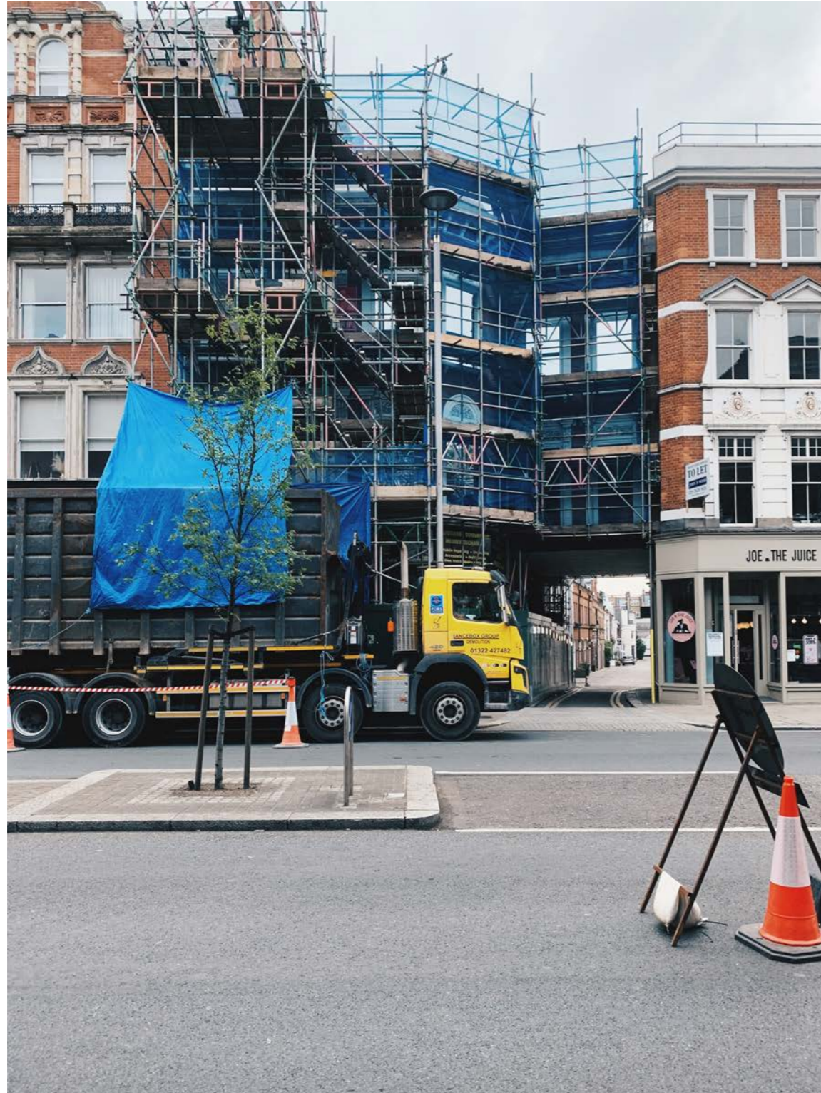
Currently, the building is being renovated on the upper floor residential units.
