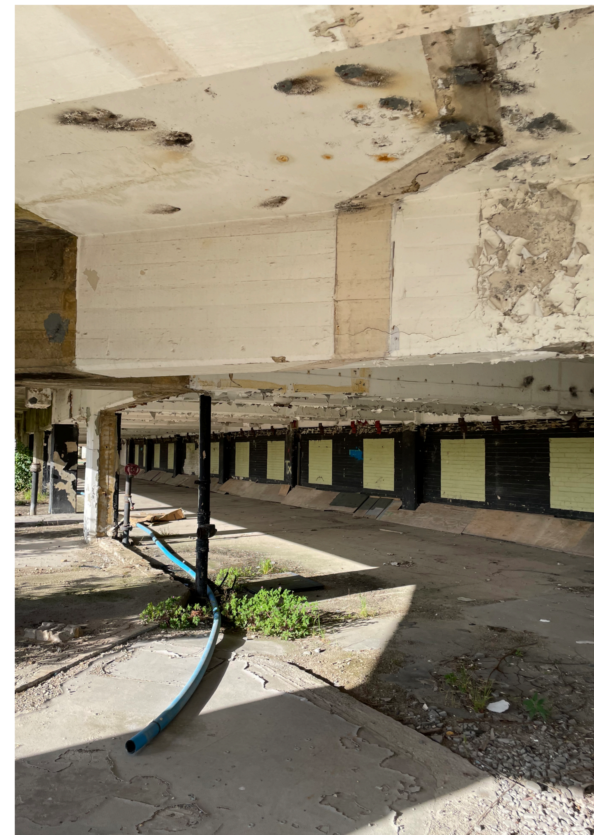
SITE EXPERIENCE: Little greenery to enjoy on site
