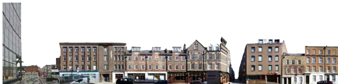
👁️ 1 PANORAMIC PHOTO LOOKING NORTH
