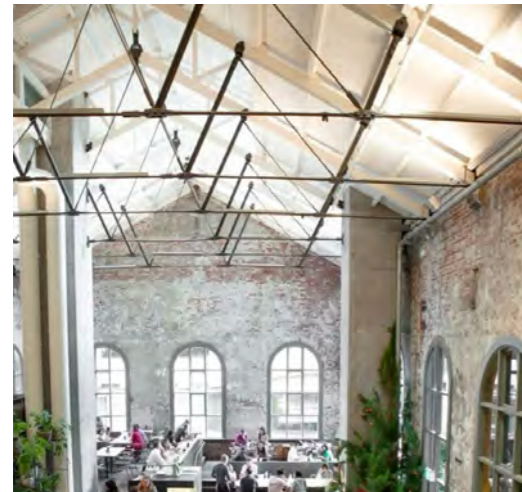
New roof with old walls
