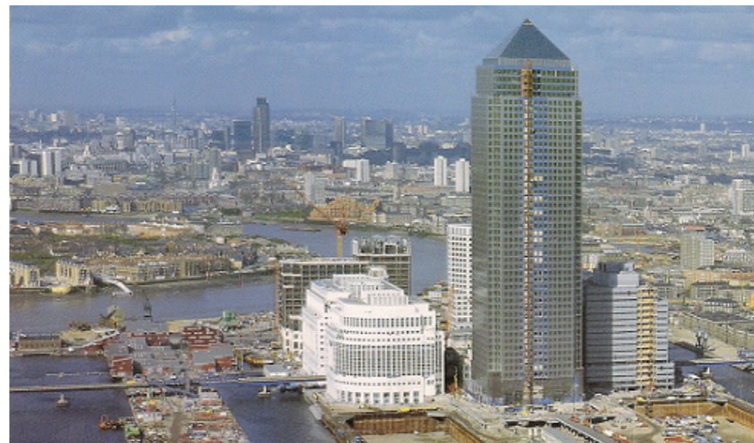
One Canada Square Under Construction, 1990s
