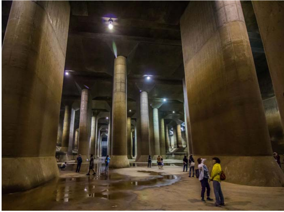
Underground Discharge Channel – Saitama, Japan
