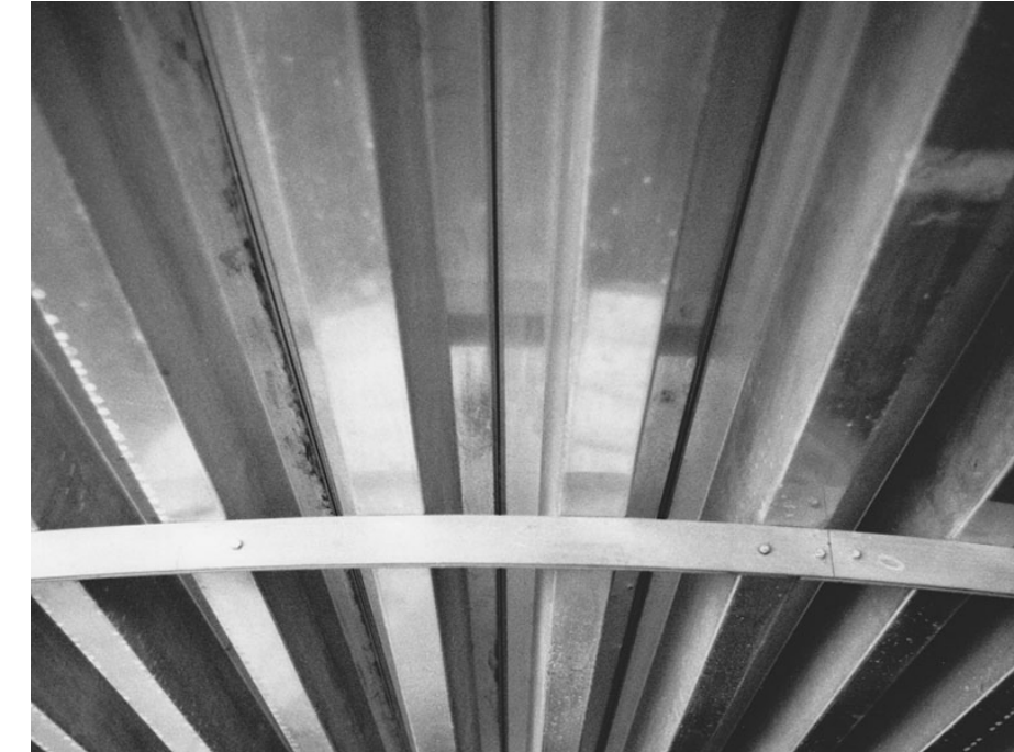
Aluminum floor joists in Dymaxion House
