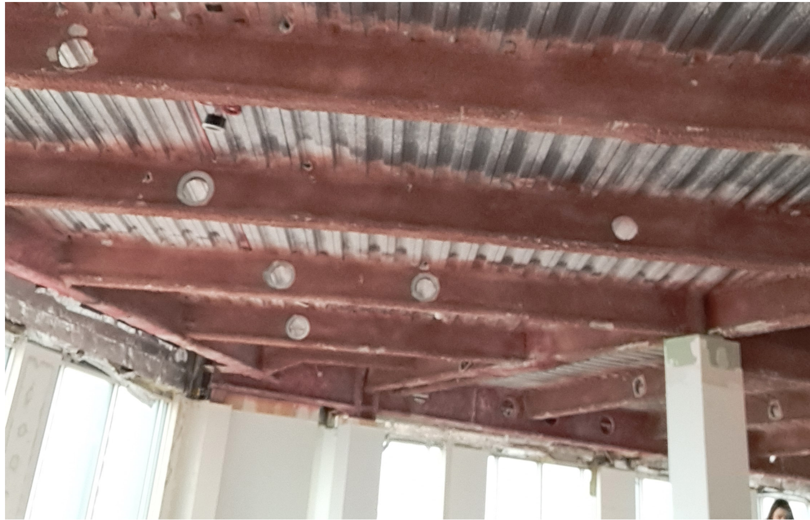
Ceiling and the structural steel of the 15 Westferry Circus building
