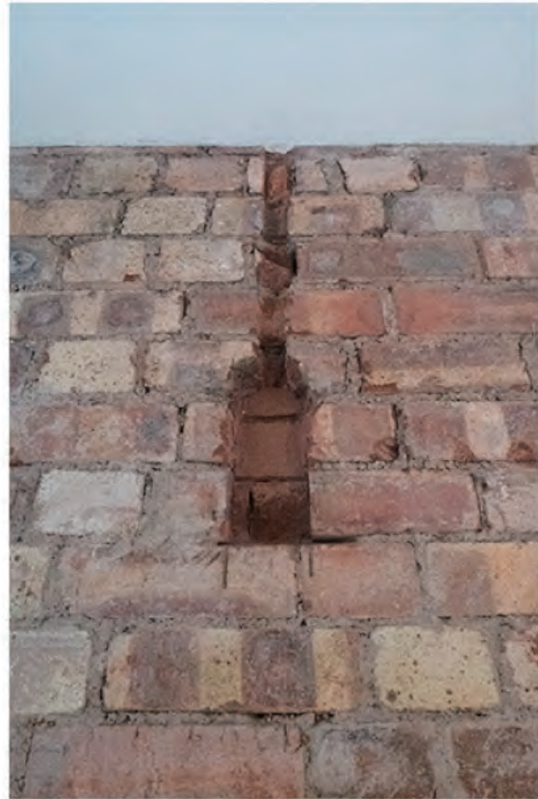
2F of site building
