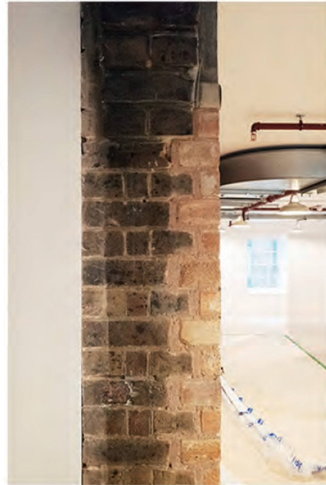
2F of site building
