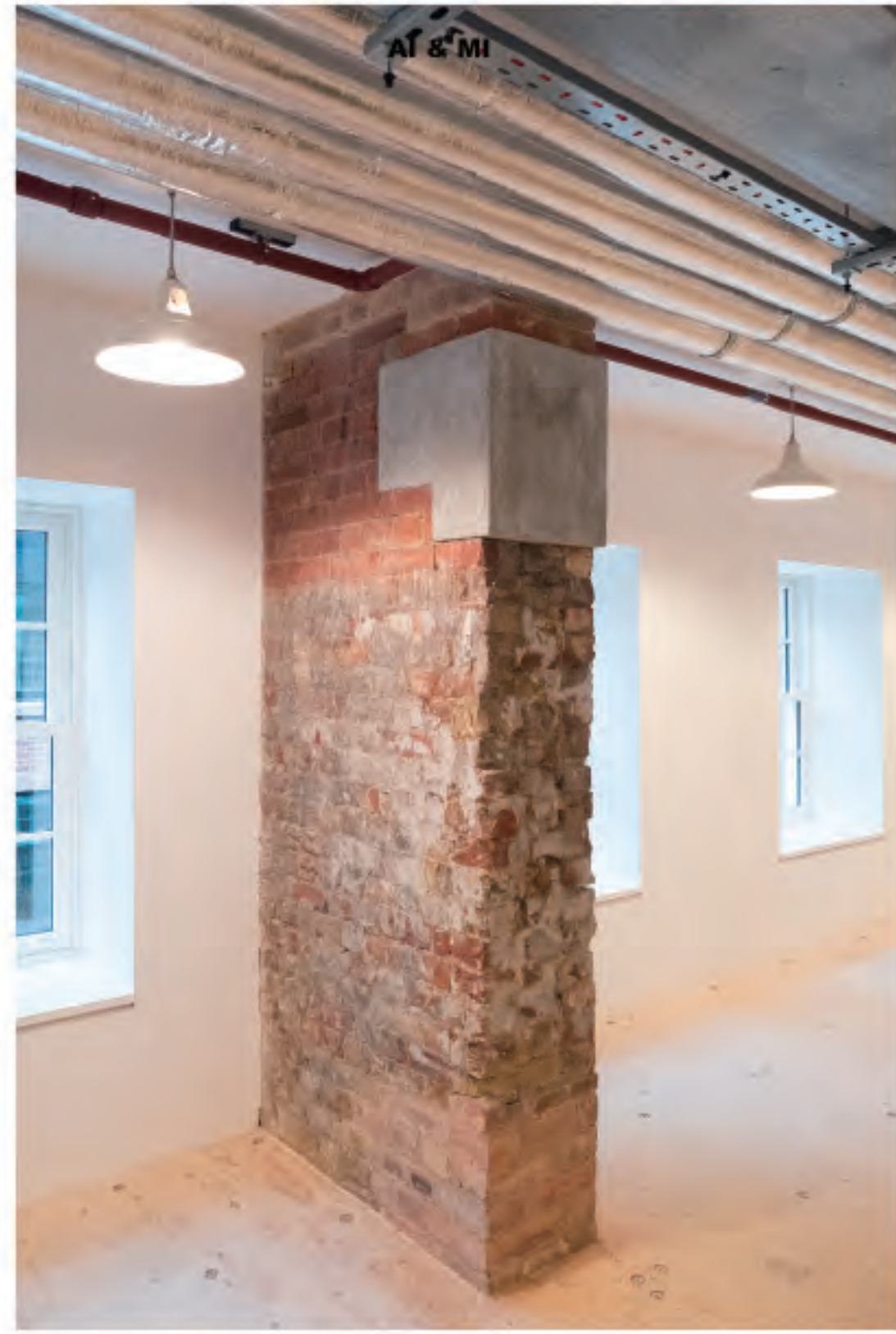
2F of site building
