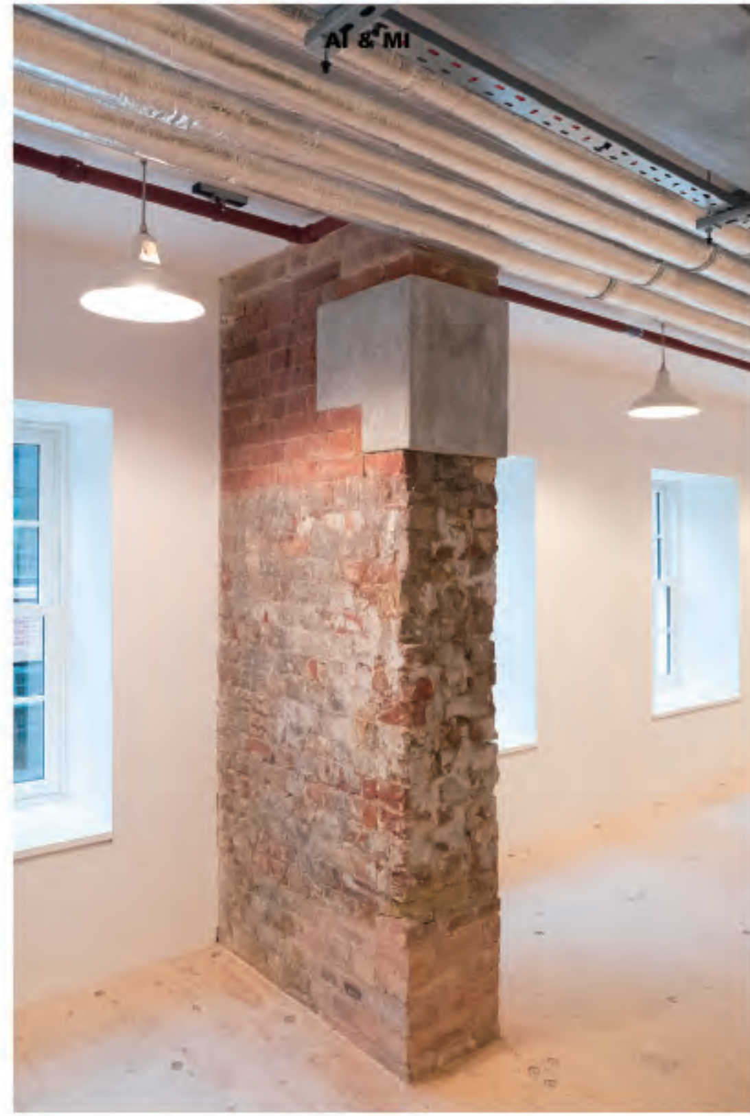
2F of site building
