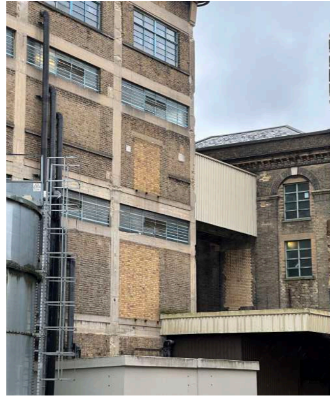
A bridge connecting 23-24 Gilldender Street, where the bridge is really dark without light. It is new added bridge compare to the Victorian style.
