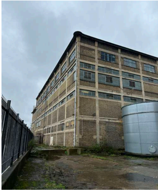
View towards the outside facade of 24 Gillender Street, a water tank is located on the outdoor space.
