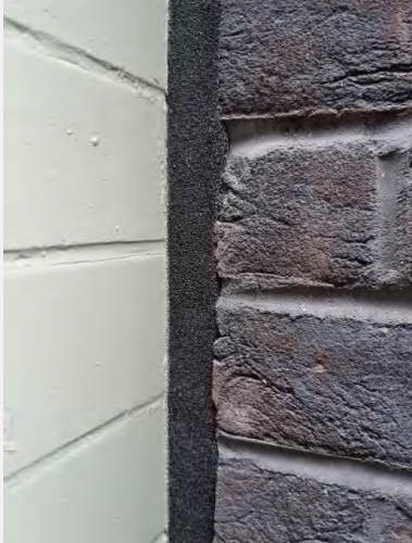
movement joint expansion joint
