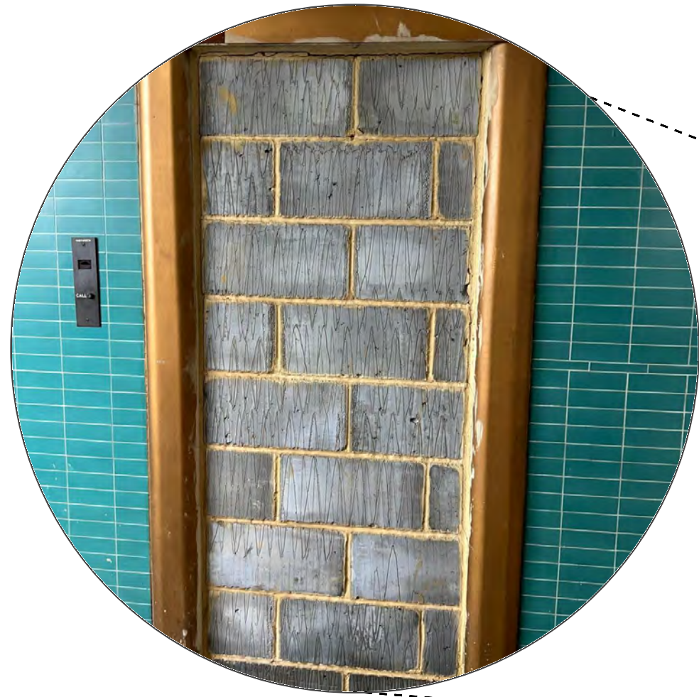
FORMER ELEVATOR SHAFT
