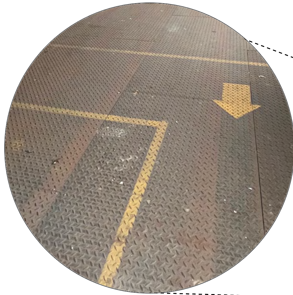
EXISTING STEEL MEZZANINE
