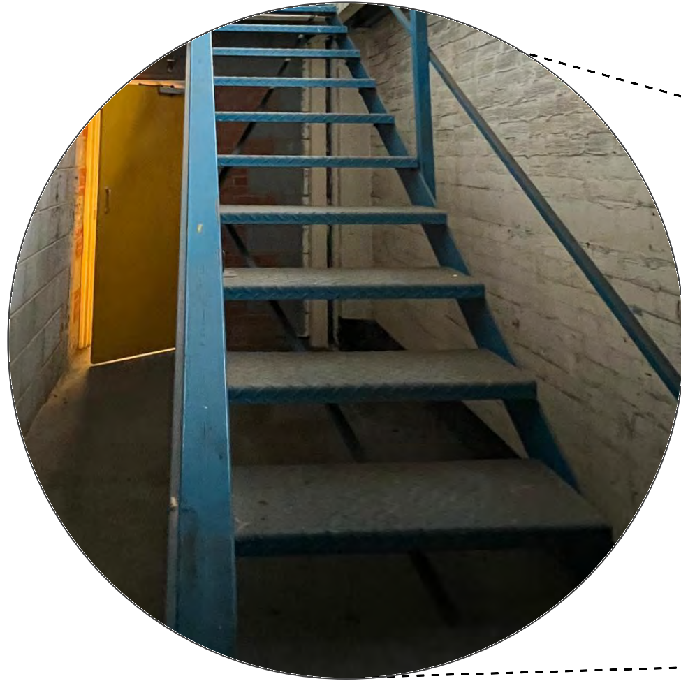
EXISTING STEEL STAIRCASE
