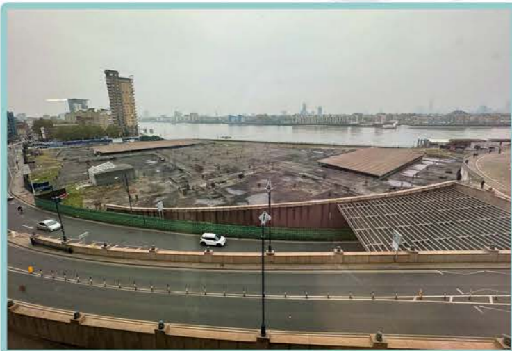
The void between the building and river
