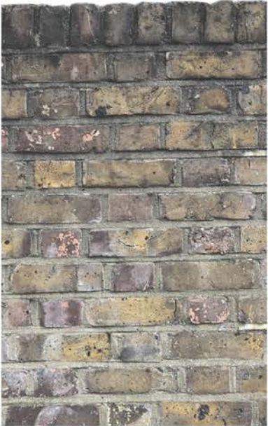
PORCHESTER TERRACE / FLEMISH BOND
